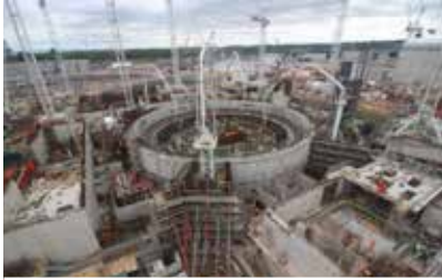
Hinkley Point C Nuclear Power Station, United Kingdom
