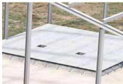
Crack inducer for industrial floors
